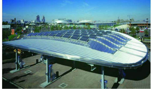
FIGURE 2: LARGE-SCALE PV INSTALLATION (SOURCE – SOLAR CENTURY)
