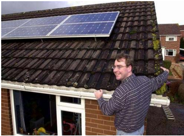
FIGURE 3: DOMESTIC SOLAR PV (SOURCE - SOLAR CENTURY)
